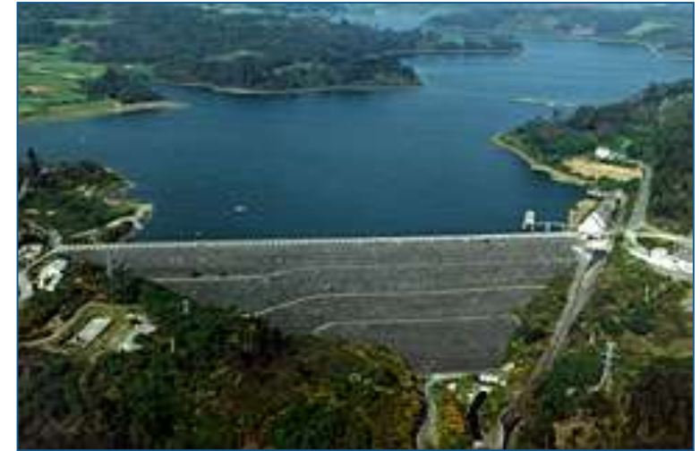
Portomouros hydroelectric dam.
