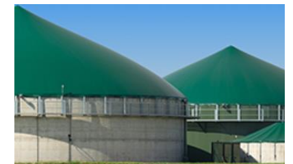
Biogas power generation
